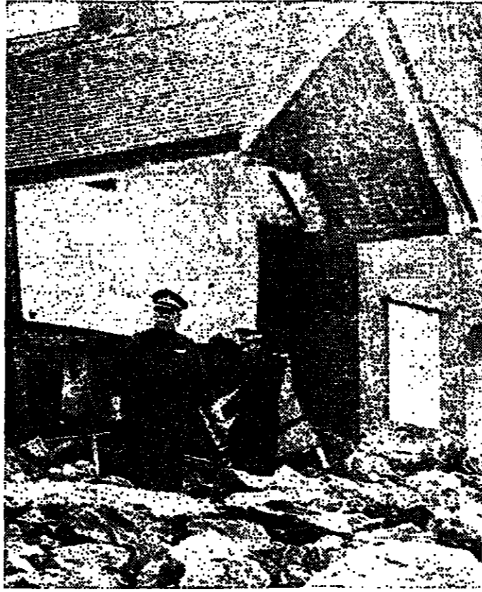
Recent storm damage at Torcross, Devon
